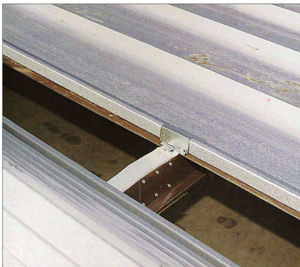
5 Concealed fastening clips secure the roof panels to the framework.
