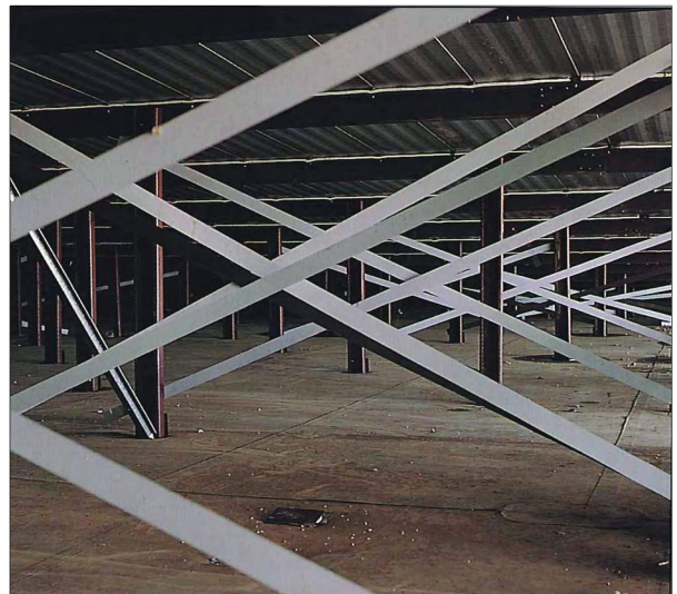
4 Cross bracing reinforces the completed framing.
