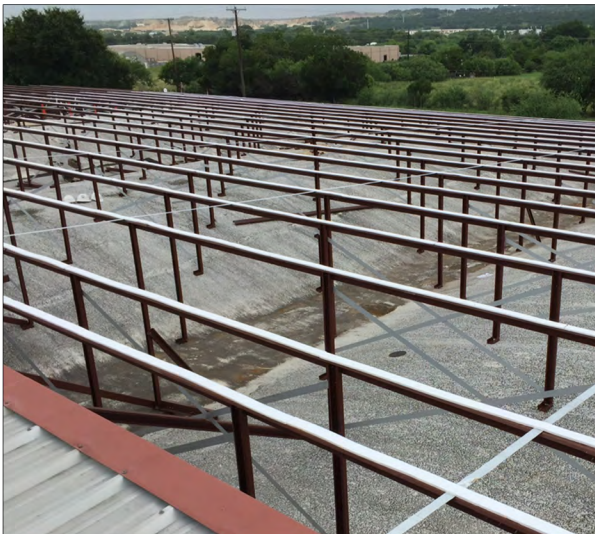
3 Zee purlins are attached to Cee channels to create desired slope.
